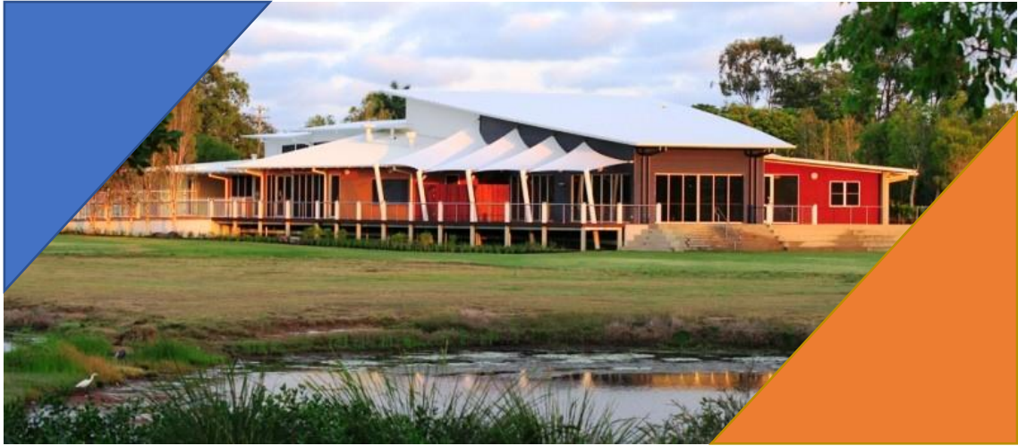
Image: Purpose built Neighbourhood Centre, Hervey Bay
